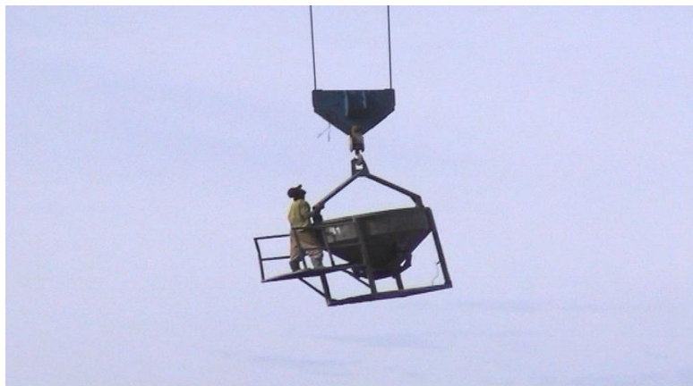
Gambar. Bucket Beton
