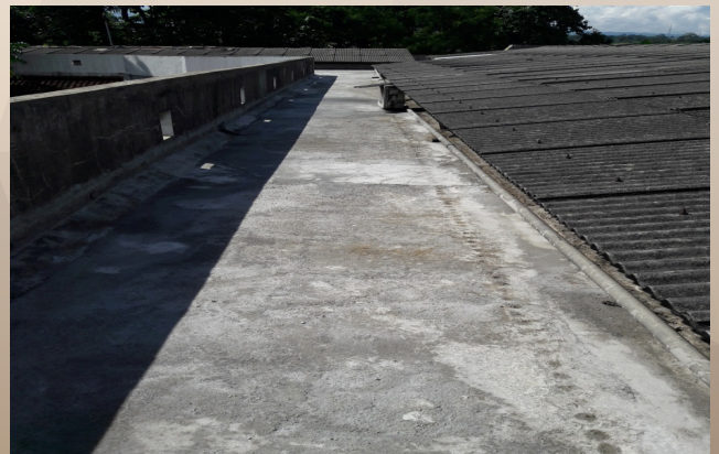
Roof construction at the main office building
