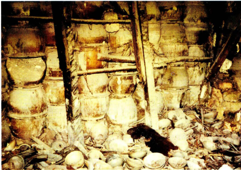
33. Dinding penguat Dragon Kiln di Singkawang, dari pasu Reinforcement wall of the dragon kiln in Singkawang consists of basins
