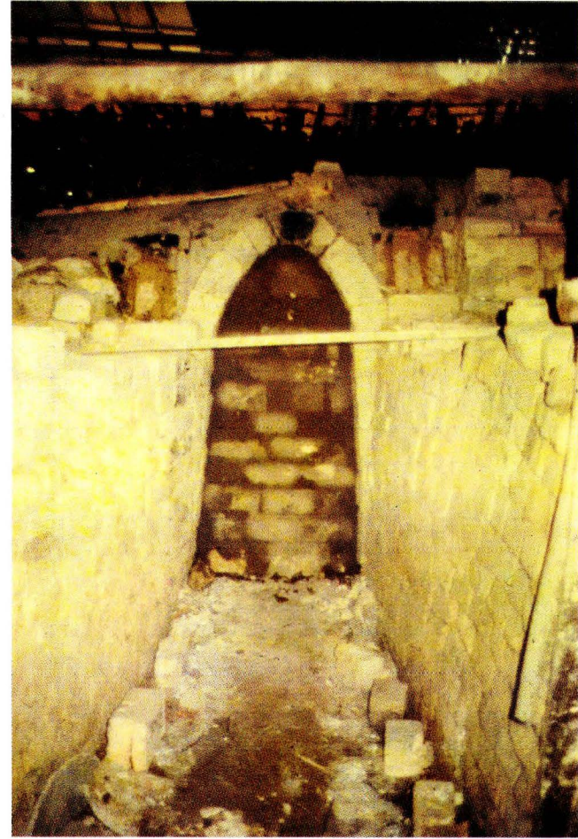
40. Bagian pintu kiln ditutup dengan bata berlepa The kiln opening is closed with mortared bricks
