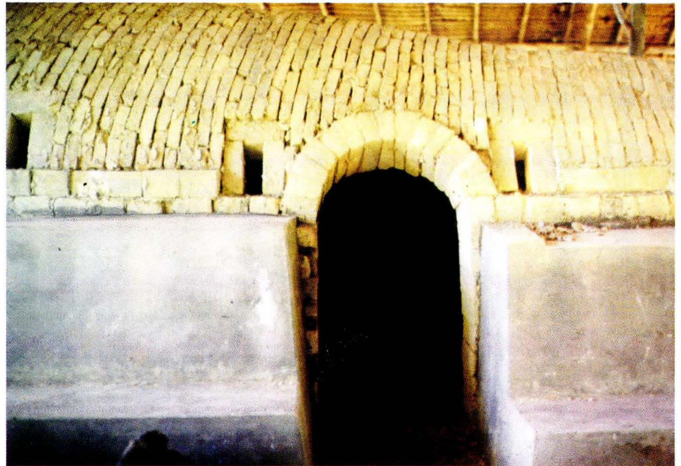
32. Bagian tungku, tampak samping. Salah satu pintu masuk ke badan tungku: Part of the kiln, side view. One of the entrances into the kiln
