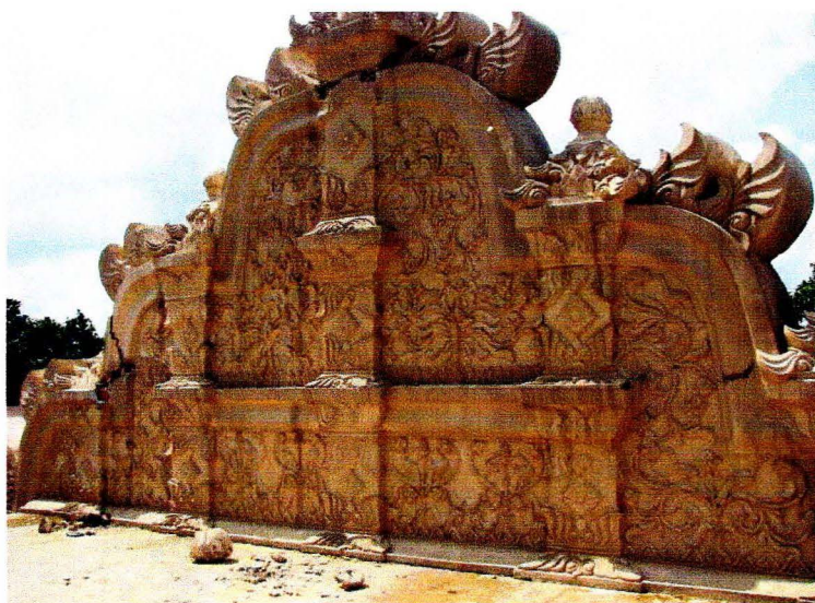
The condition of the west gapura agung before the emergency action
