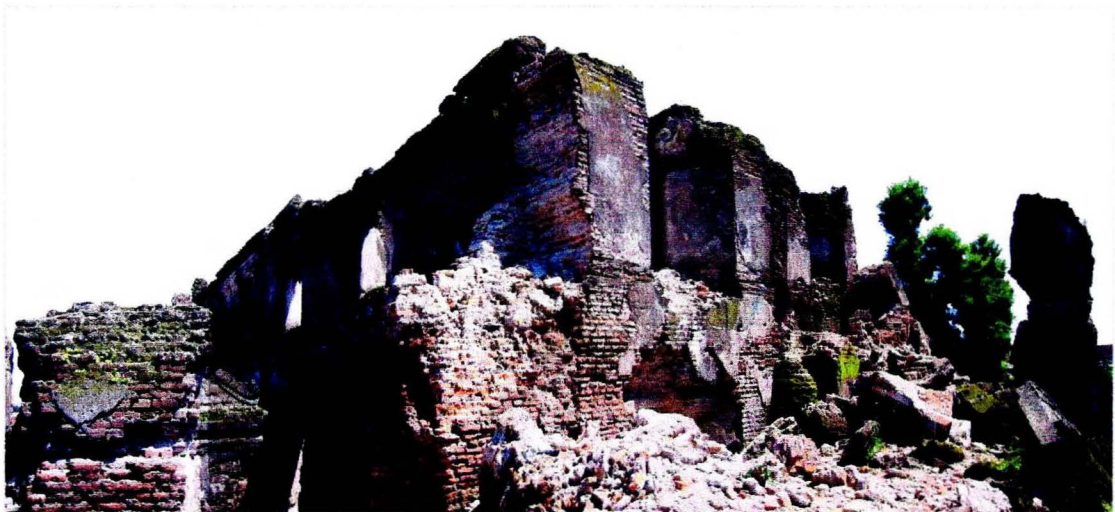
The condition of Pulo Kenanga from southwest view
