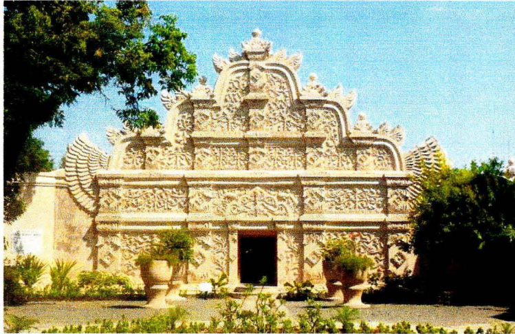
Gapura Agung before the earthquake
