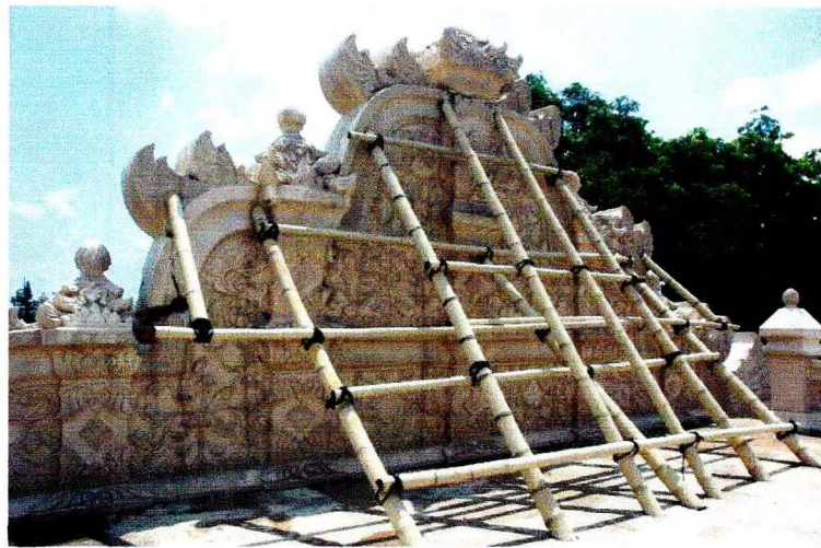
The condition of the gapura agung after the emergency action
