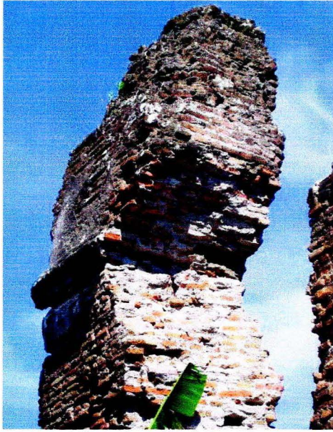
The detail of the dangerous broken structure of the remains The left picture - from outside view. The right picture – from the inside view
