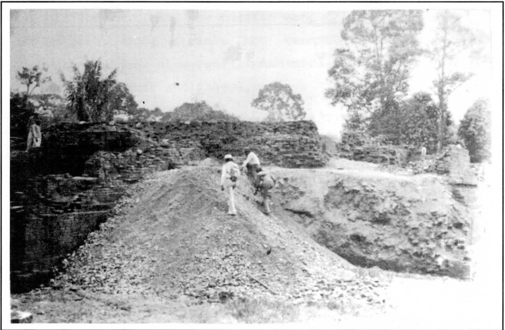
Chandi Kedaton. Part of the stones and gravel from the inside of the structure
