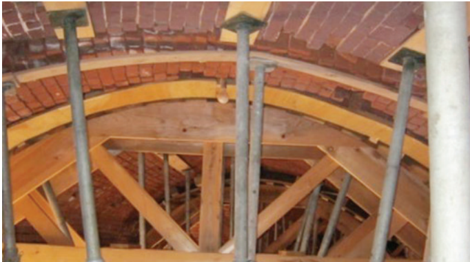
Supporting structure temporer
