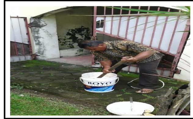
***FOTO KEGIATAN PEMBUATAN ADONAN (CAMPURAN) PLESTERAN DINDING DAN ROLLAK BANGUNAN GEDUNG K***
